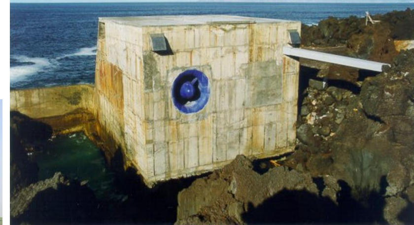
Oscillating Water Column
