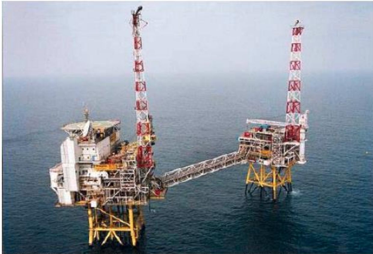
Fig. 0. The Draupner S and Draupner E platforms in the North Sea, Photo: Øyvind Hagen, Statoil.
